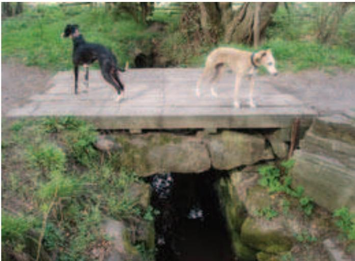
The old bridge over Arrove Brook where it turns towards Arrove Park. One of the original stone slabs can still be seen, now badly cracked. For many years, thick wooden planks have been used to safely span the brook.
