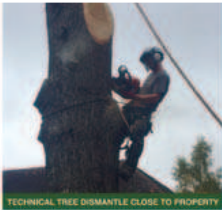
TECHNICAL TREE DISMANTLE CLOSE TO PROPERTY
