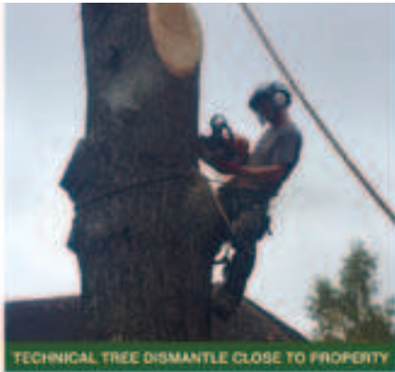
TECHNICAL TREE DISMANTLE CLOSE TO PROPERTY
